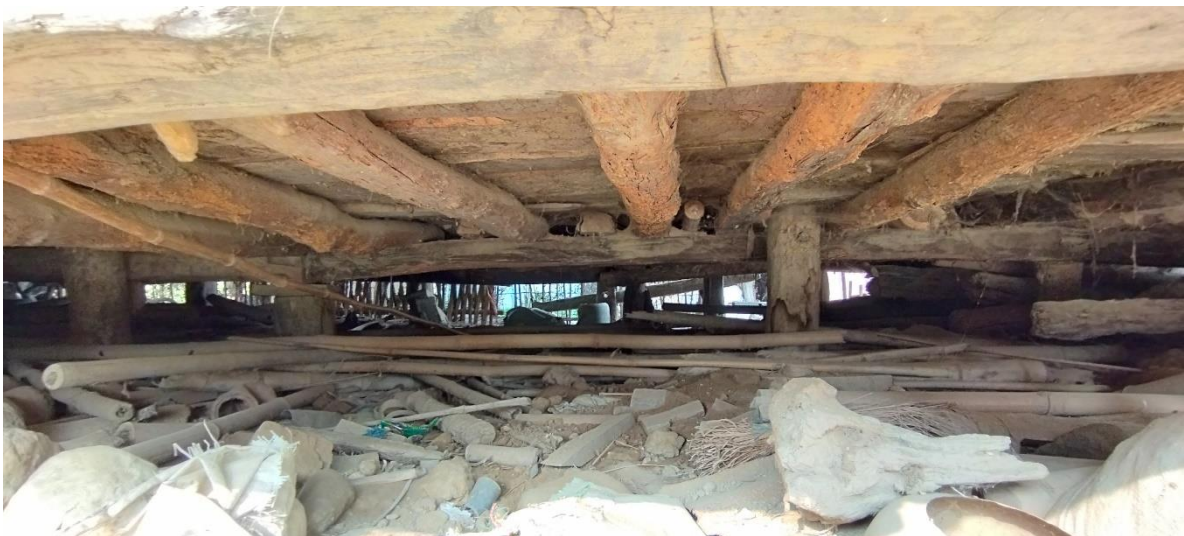
Figure 7 beams of the raised ground floor in plinth
