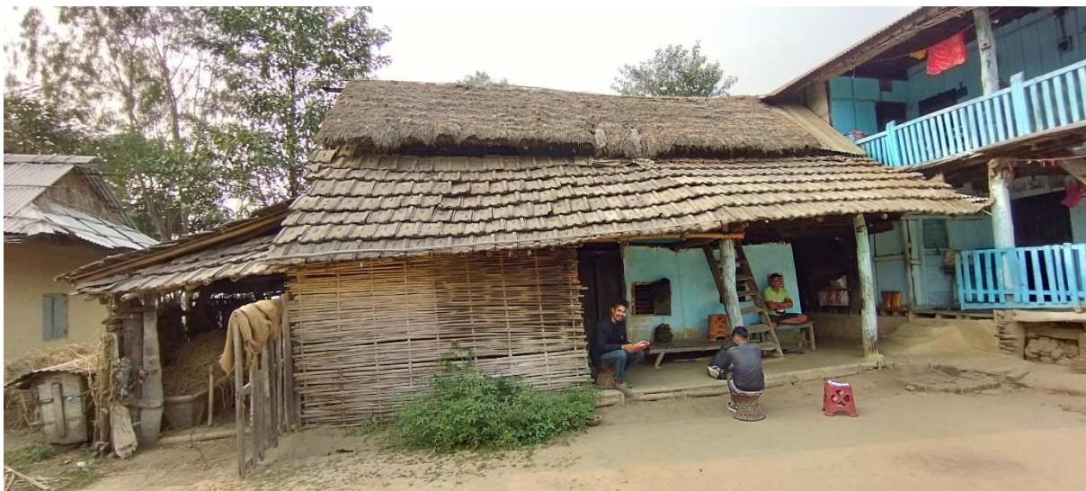
Figure 9 Roofing of the store house with clay tiles and straw bale
